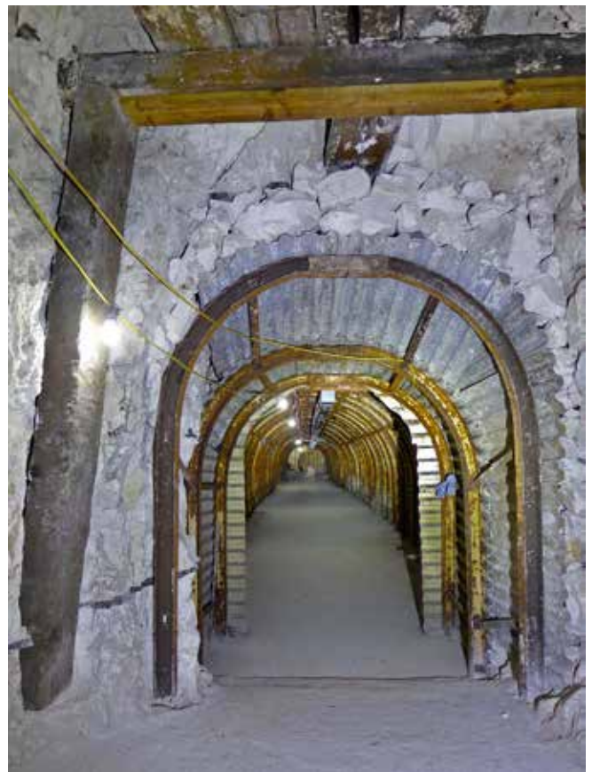
Tunnel construction techniques: removal of steelwork is ill-advised! Photo Tim Wellburn
